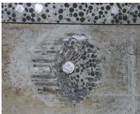
Dismantled shear fracture of a light weight concrete dowel
