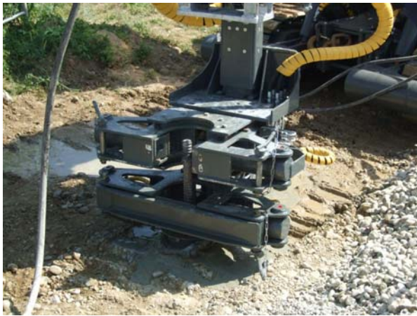
Picture: 11 Installation of micro-piles
