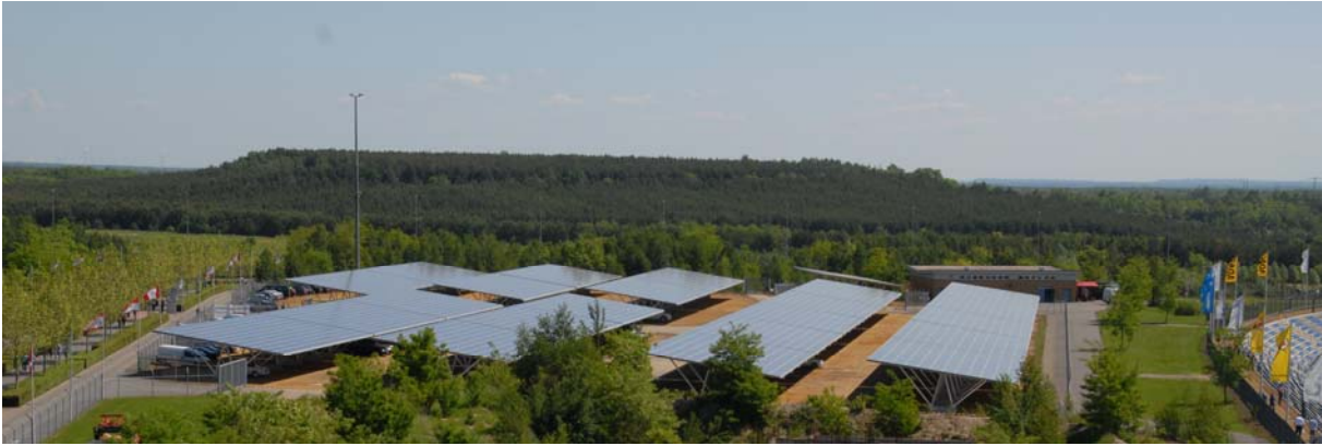
Picture 13: Carport plant with a performance of 1 MWp close to the Lausitzring
