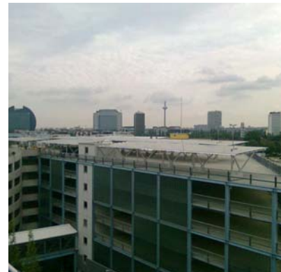
Special project on a parking deck
