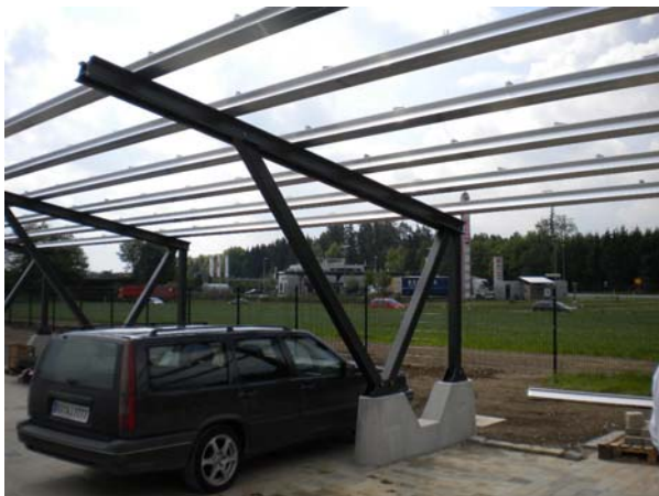
Picture 5: Concrete foundation as a vehicle impact protection Picture 6: Precast concrete part connection detail
