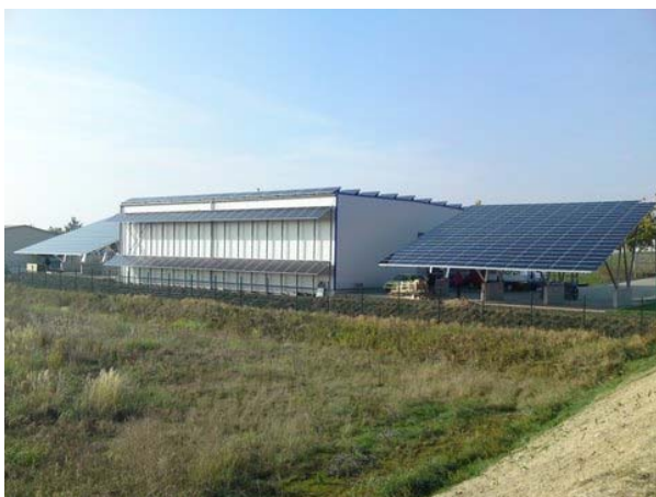
Picture 7: Carports with an inclination of 25°
