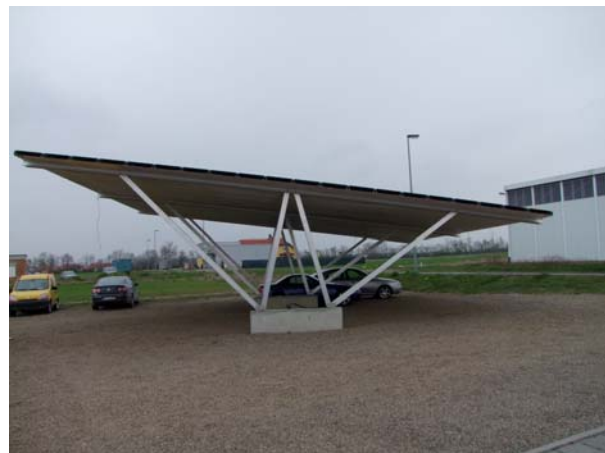
Picture 8: Carport with an inclination of 10°
