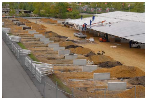
Picture 10: Surface foundation (new foundation)
