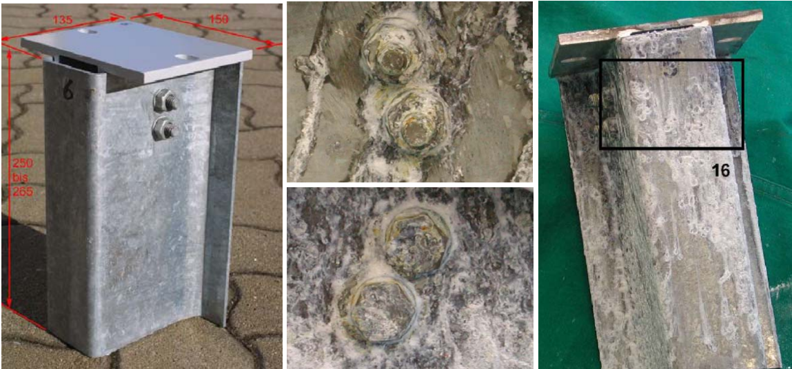
Figure 5: Material selection regarding high-grade steel in relation to the risk of corrosion
