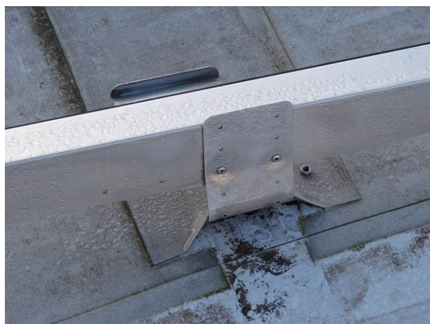
Figure 7 Local detachment of the glued lug due to peeling
