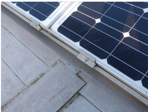
Figure 1 Fastening with glued lugs on membrane
