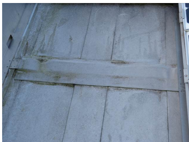
Figure 5 Glued lugs over connection sheets
