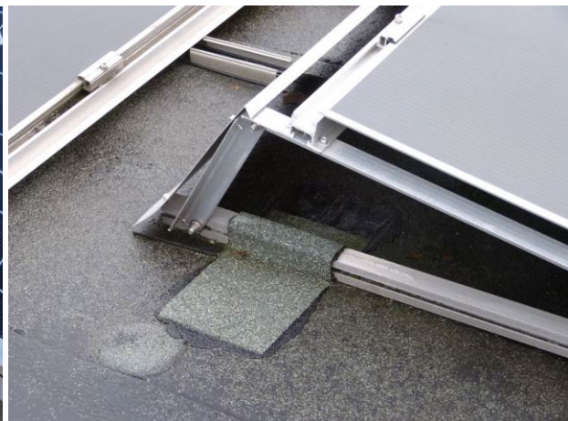
Figure 2 Fastening with welded lugs on bitumen
